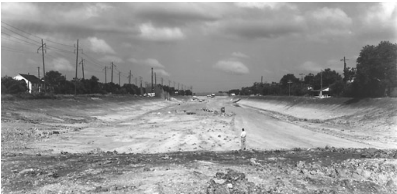
Excavation: This view dating from around 1960 shows the excavation for the depressed section of freeway near downtown. At the time, this excavation for the 10-lane freeway was the largest and most impressive construction project to occur on Houston's freeway system. (Photo: HMRC MSS 334-1153)
