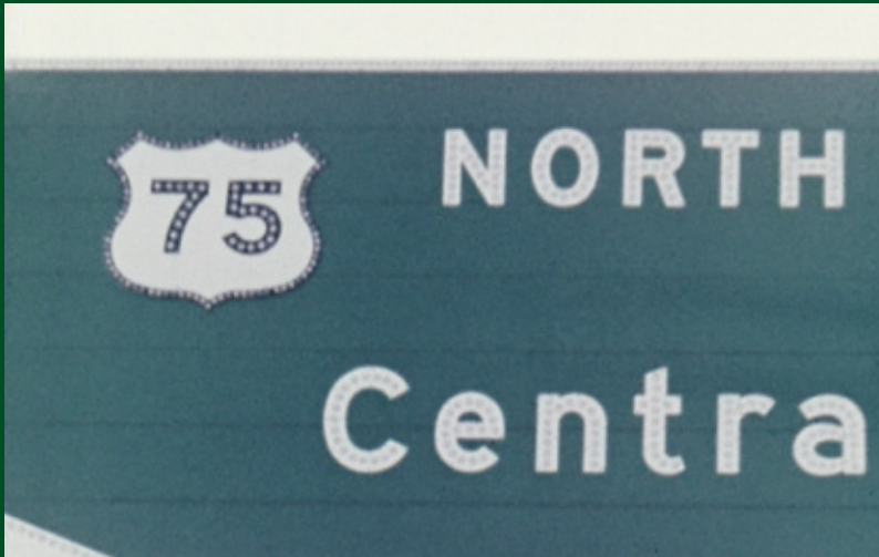
#15: This view shows a guide sign to Central Expressway with "button copy" on the lettering and outlines. Button copy placed small reflectors along the paths of letters and outlines to illuminate those features. It was typically used on signs which did not have independent lighting. Today, freeway guide signs are made of highly reflective material which is brightly visible from automobile headlights alone, eliminating the need for sign lighting or button copy.
