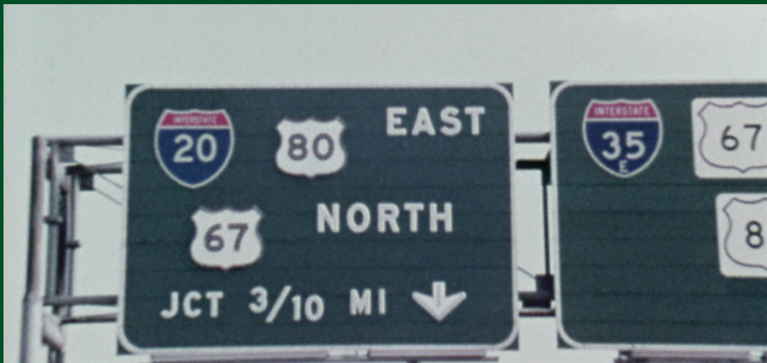
#14: This image shows the most interesting artifact—the IH 35E shield. Notice that there is a very small “E” beneath the “35” number. Modern signs have the “E” immediately to the right of the “35” in the same font size as the numbers.
