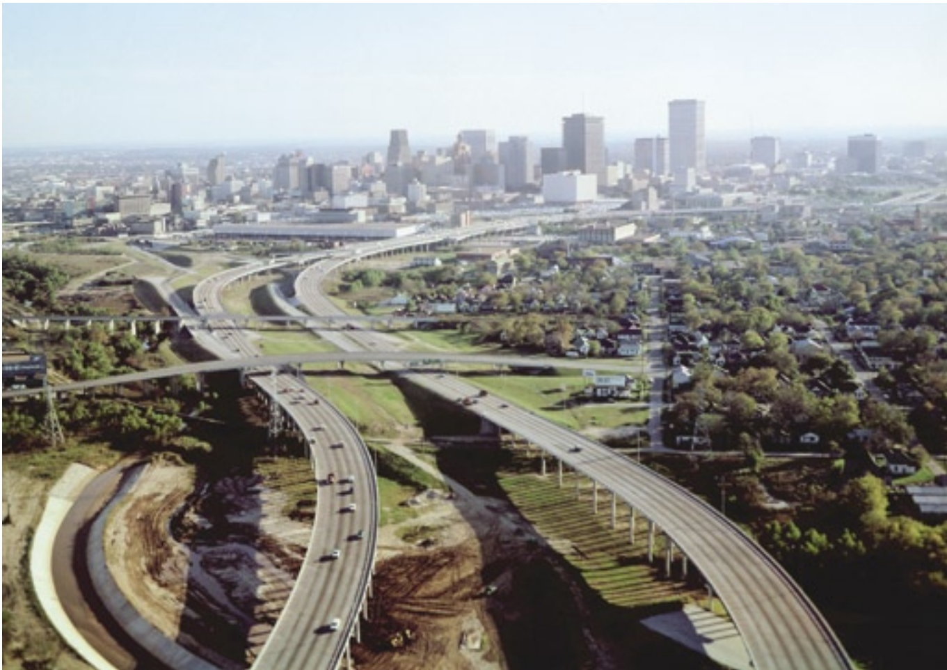
One freeway complete, one to come: These views show the IH 45-IH 10 multiplex interchange prior to the construction of IH 10. The wide median and adjacent cleared right-of-way would later become IH 10 and its connection ramps. The upper photo was taken just after the freeway opening in July 1962. The lower photo was taken in December 1964. (Photos: upper, HMRC MSS 157-907; lower, TxDOT)
