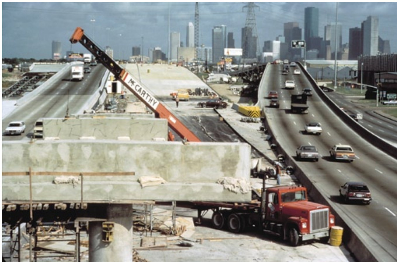
Houston's freeways turn into an obstacle course: The reconstruction and expansion program got underway in the early 1980s and launched the seemingly never-ending era of construction detours on Houston's freeways. This July 1985 view shows the Gulf Freeway at Lockwood, with northbound traffic diverted to an adjacent structure. On the other side of this overpass was the notorious "S" curve detour. The Gulf Freeway was Houston's first freeway to undergo a comprehensive rehabilitation with a fully integrated bus transitway. (Photo: Chuck Fuhs)
