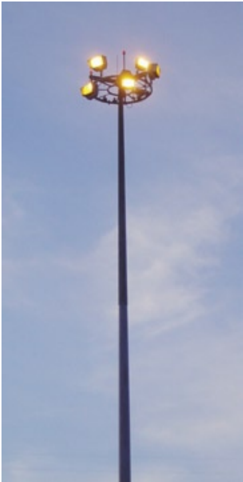
Lighting the freeways, not the sky: The left photo shows a typical high mast equipped with directed floodlights. Floodlights were used for the Z-pattern high mast illumination that was standard in Houston's first generation of high mast lighting. The floodlights were difficult to aim and had the potential to send light upwards into the atmosphere, contributing to the sky glow effect. Starting in the early 1990s, TxDOT began to use a ring of cutoff light fixtures that point toward the ground. The right image shows the arrangement of lights that is now standard for new installations of high mast lighting on Houston freeways. (Photos: July 2002)
