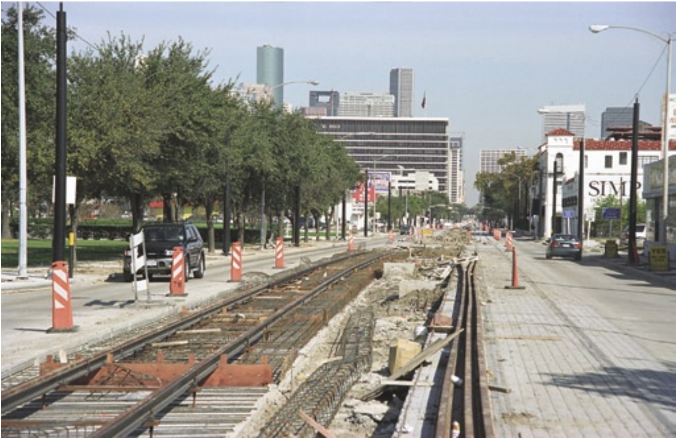
Streetcars return to Houston: After a 64-year absence, streetcars will return to Houston streets in 2004 on the $325 million, 7.5-mile (12 km) light rail line. Construction began in 2001 after substantial controversy and litigation. This photo shows tracks being laid south of downtown on Main Street. (Photo: November 2002)
