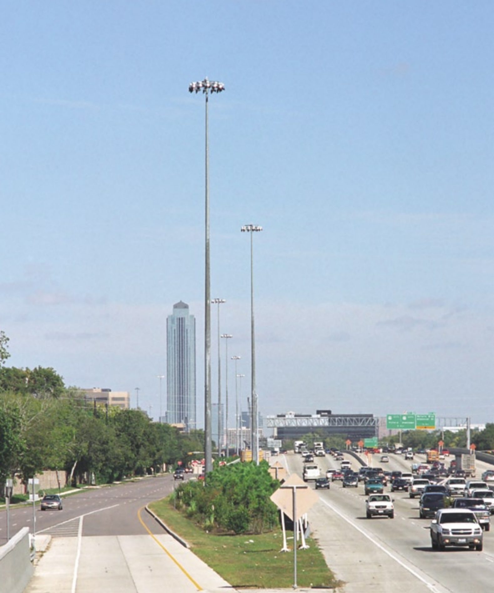
Houston—high mast illumination capital of America: This view of high mast light fixtures lined up along the West Loop in Bellaire is typical of most Houston freeways. Houston makes extensive use of high mast illumination along linear sections of freeway—probably more than any other place in the world. (Photo: November 2002)
