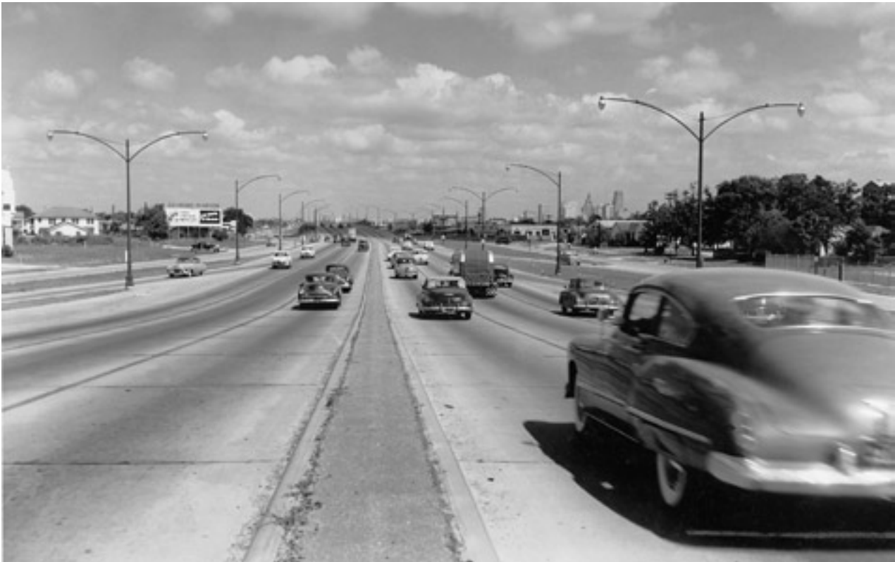
The first generation freeway: This view of the Gulf Freeway shortly after its completion demonstrates two of the shortcomings of the first generation freeway: lack of a central guardrail and light fixtures placed close to the main lanes with no protective guardrail. Other shortcomings were short merging distances at on-ramps, poor geometrics, roller-coaster grades, and traffic-carrying capacity designed to meet forecasts that were much too low. (Photo: TxDOT)
