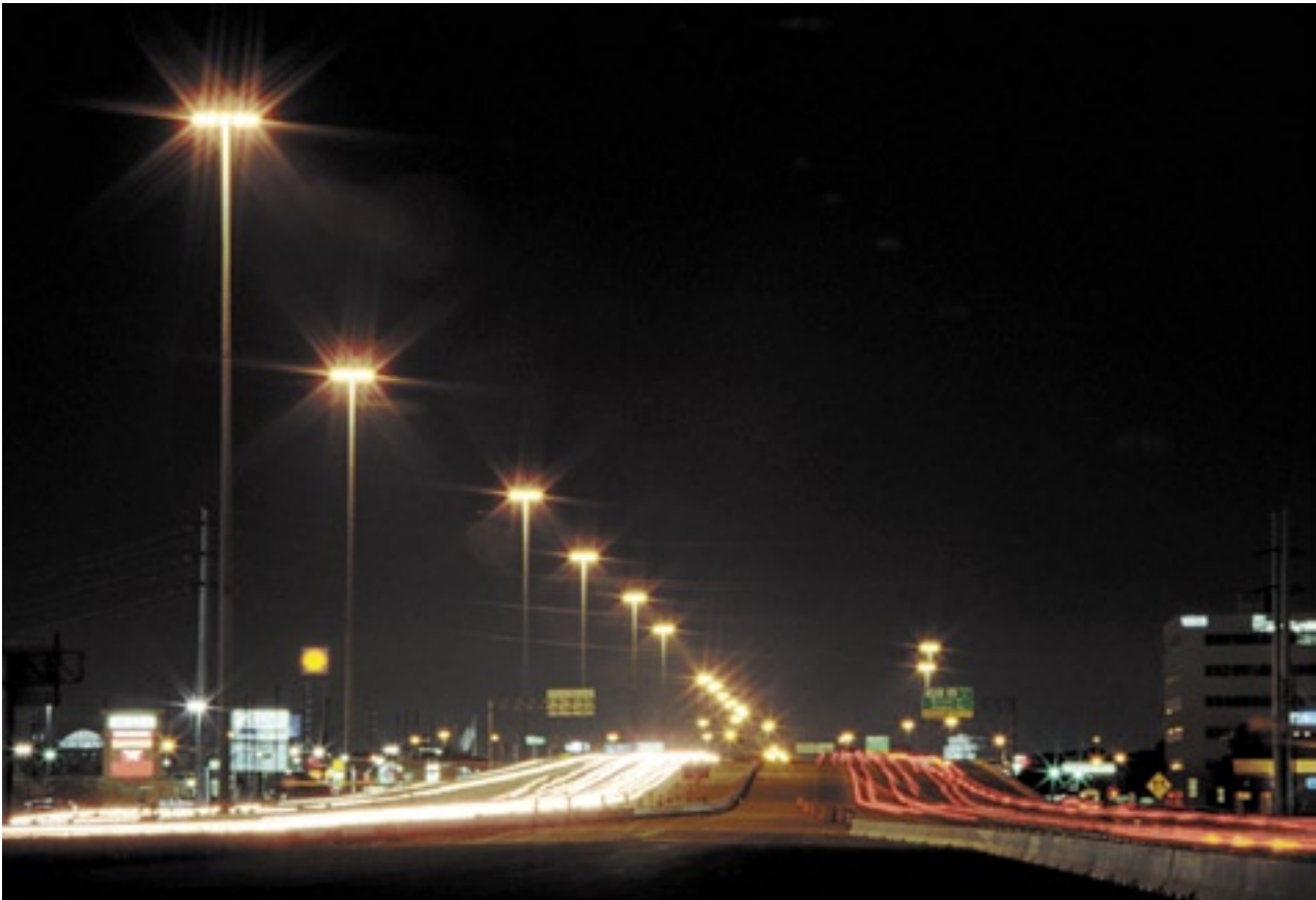
Cutoff high mast lighting: These masts on the Southwest Freeway north of Sugar Land use cutoff light fixtures. (Photo: June 2002)
