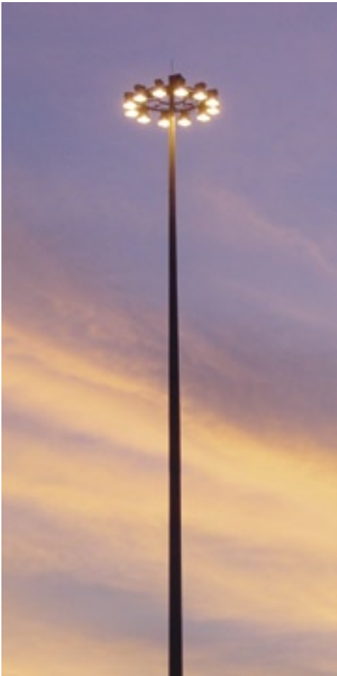
Lighting the freeways, not the sky: The left photo shows a typical high mast equipped with directed floodlights. Floodlights were used for the Z-pattern high mast illumination that was standard in Houston's first generation of high mast lighting. The floodlights were difficult to aim and had the potential to send light upwards into the atmosphere, contributing to the sky glow effect. Starting in the early 1990s, TxDOT began to use a ring of cutoff light fixtures that point toward the ground. The right image shows the arrangement of lights that is now standard for new installations of high mast lighting on Houston freeways. (Photos: July 2002)
